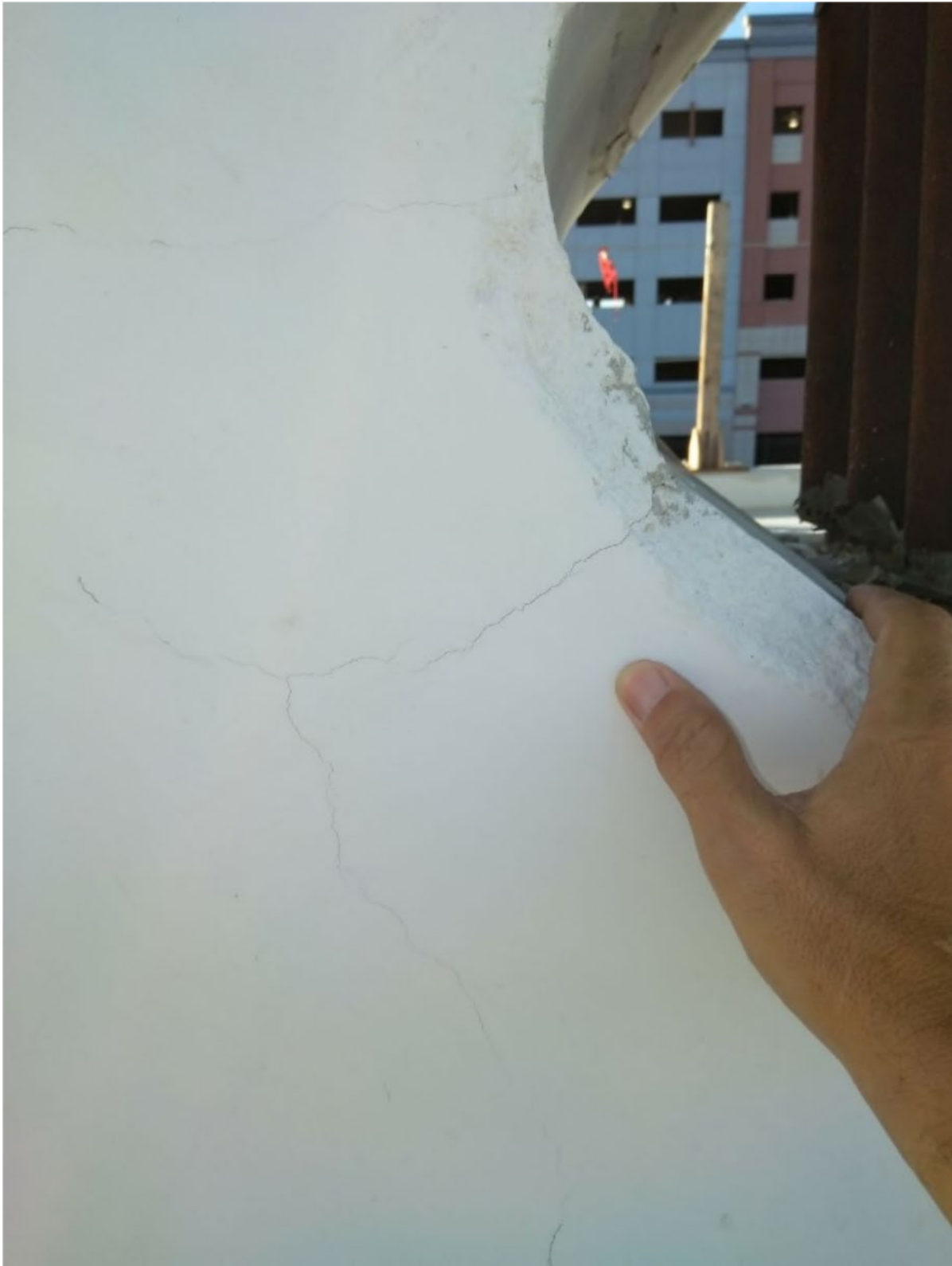
Figure 16 Photo #2 in 2/28/2018 E-mail from MCM to FIGG
