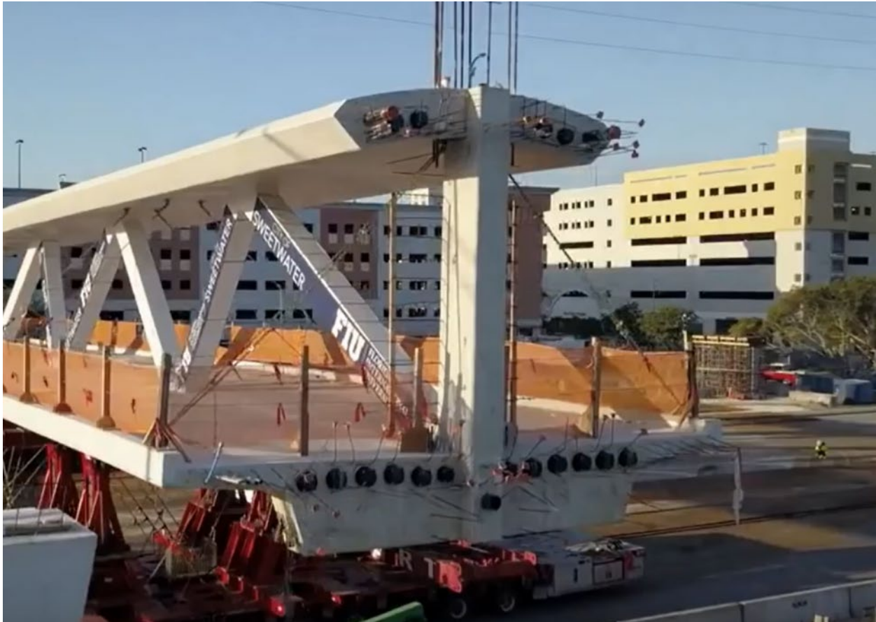
Figure 22 North end of the main span truss during transportation, generally free of cracks
