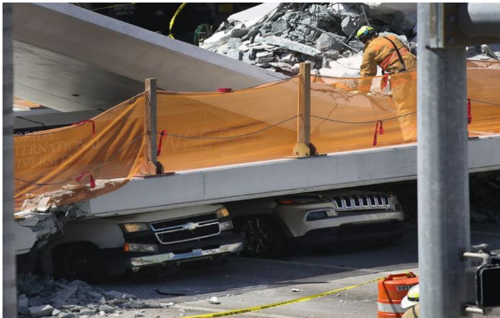
Figure 75 Vehicles crushed by falling bridge
