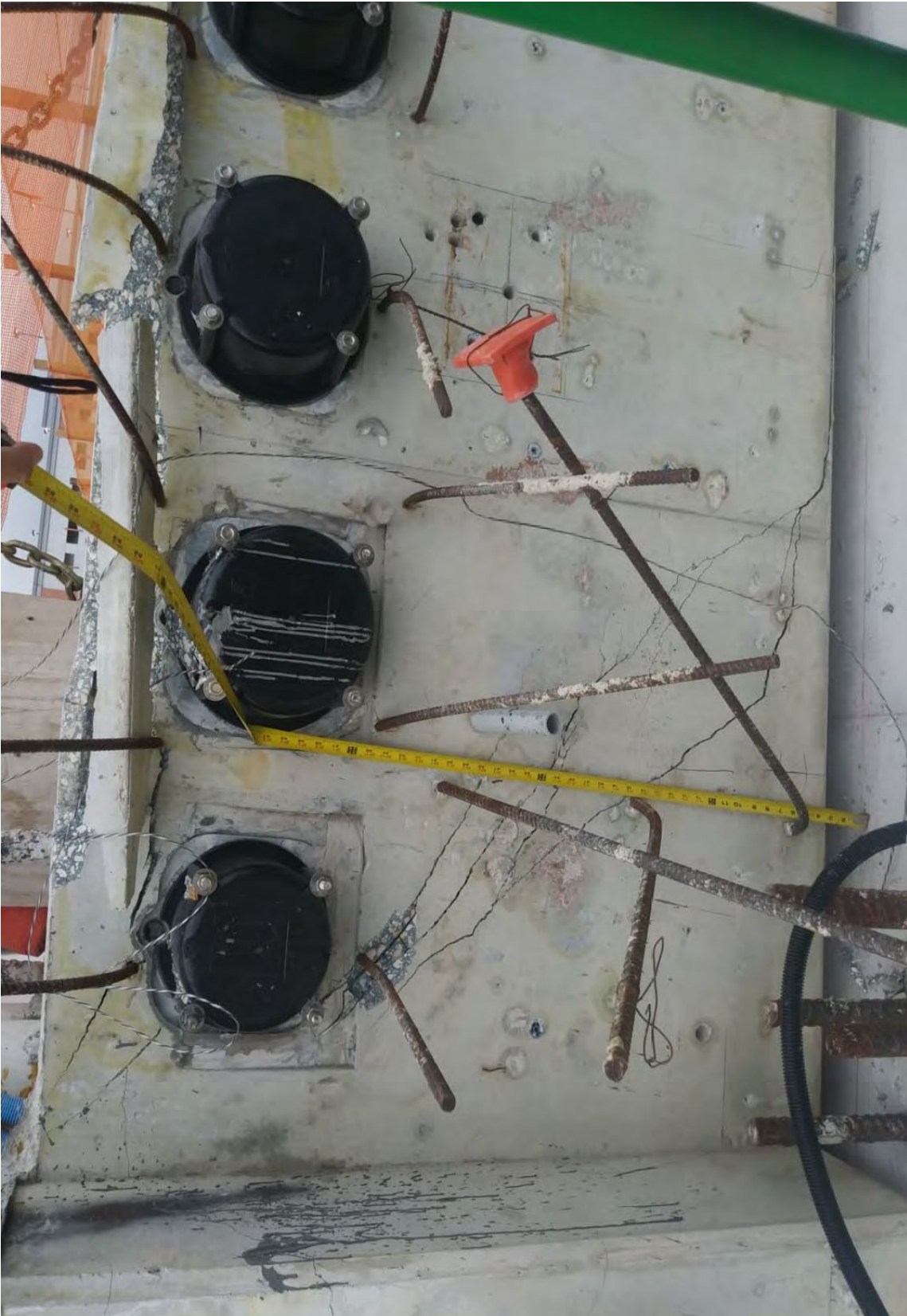
Figure 25 Cracks at the west side diaphragm II MCM email of 3/12/2018, by BPA – side face
