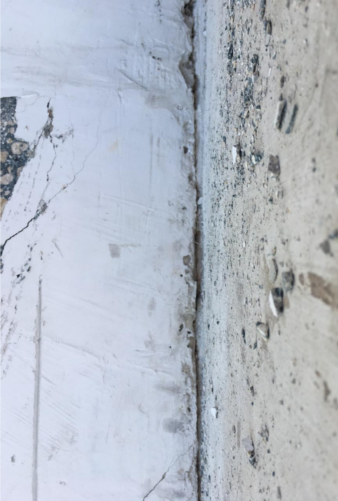
Figure 37 Cracks at the construction joint of the main span deck and diagonal 11 on 3/13/2018 by BPA
